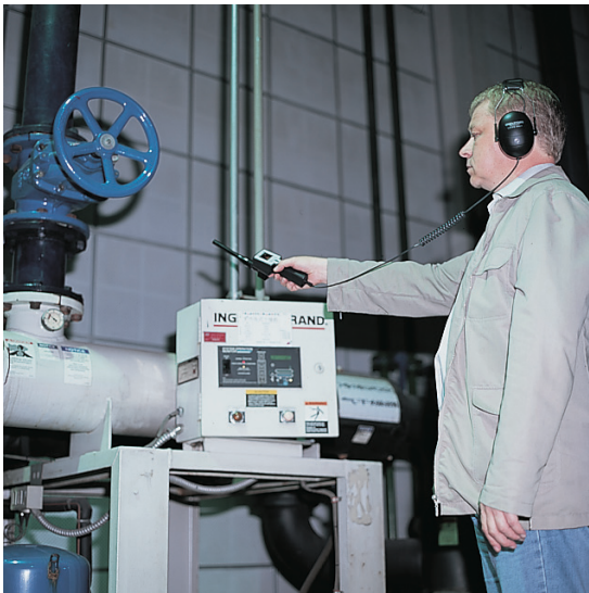
Leak detection with focus tube
