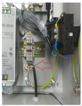
The power cable for the 230VAC is connected to the terminals inside of the cabinet as shown in the picture on the left.
